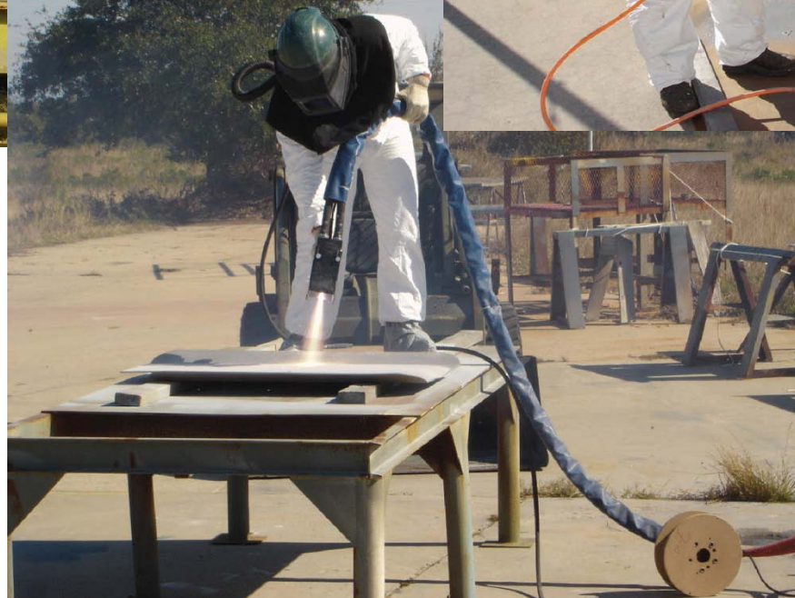
Depaint with Blast Recovery System (BRS)
